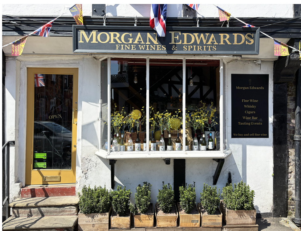
The building is Grade II listed
